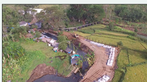
2 Jalur Pipa Intake (SPAM Umbulan)
